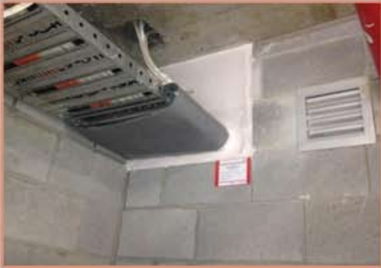
TBA Firefly Intubatt Seal with Tray and Cables FRL-/120/120
