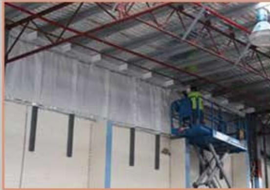
TBA Firefly Titan to the Head of External Wall FRL 60/60/60
