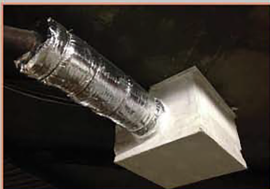
TBA Firefly Intubatt Boxout/Bulkhead with Copper Pipe FRL-/120/120
