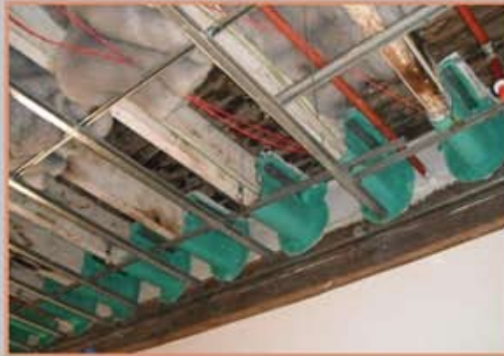
TBA Firefly Linear Gap Seals to the Head of wall using Intubatt then timbers protected using Timber Penowrap System.
