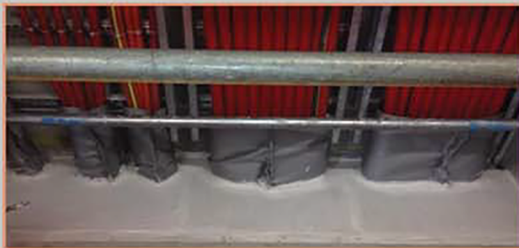
TBA Firefly Intubatt Floor Seal with Electrical Cables FRL-/120/120
