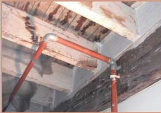
TBA Firefly Linear Gap Seals to the Head of wall using Intubatt then timbers protected using Timber Penowrap System.
